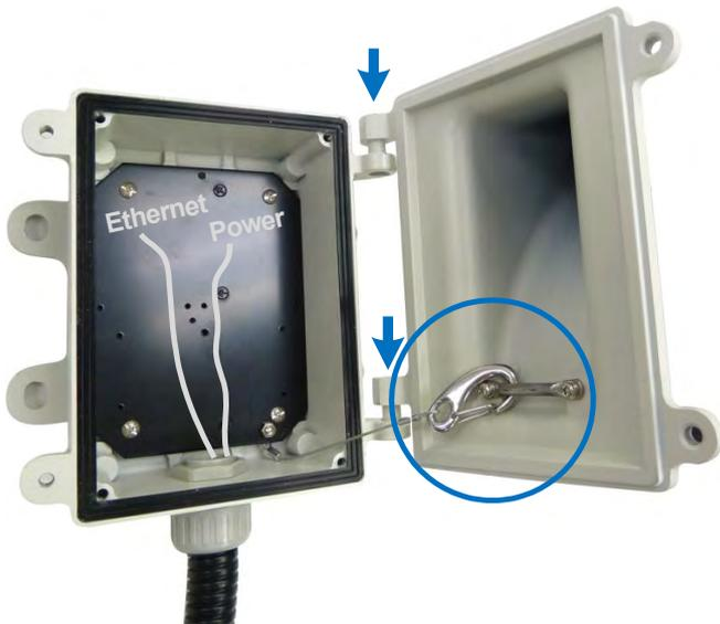
7. Connect the network, power and other cables to the camera. See *1.7 Connecting the Data Cable, GV-Fisheye IP Camera H.264 User's Manual* on the software CD.
